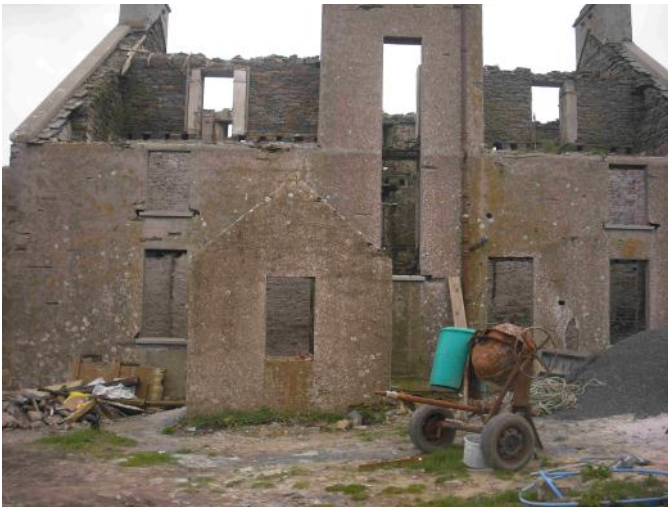
Old porch before demolition
