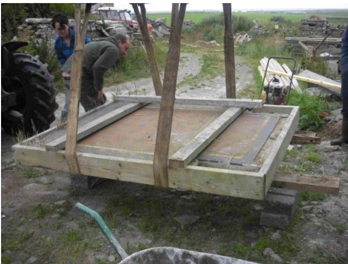
Original tiled porch floor going back in
