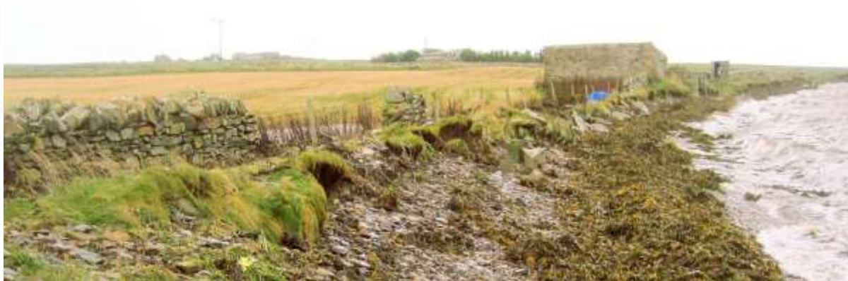
Part of the dyke below Midgarth which was destroyed by heavy seas only a few months after having been rebuilt.
