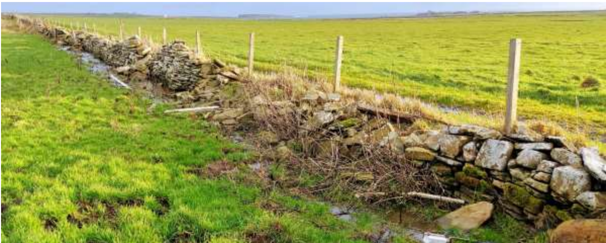
A neglected dry-stone dyke, where a few ragstones rubbed off by cattle and not replaced soon grew until the dyke is now little other than a heap of stones.
