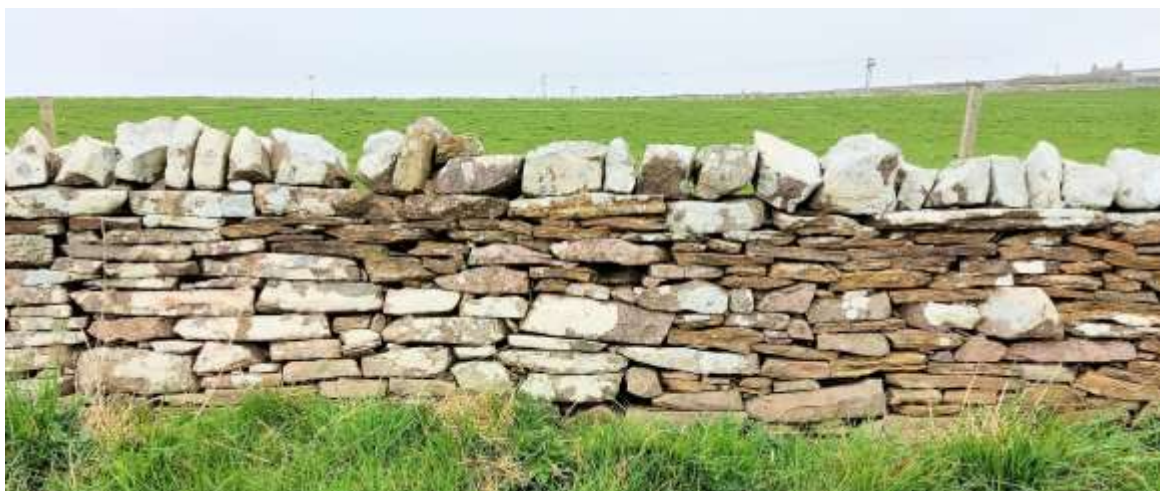
The change from red sandstone on the left to grey whinstone on the right. The whinstone is of poor quality and showing signs of erosion and splitting so may well have been among the first, softer, stones to be taken from the top layers of the quarry.
