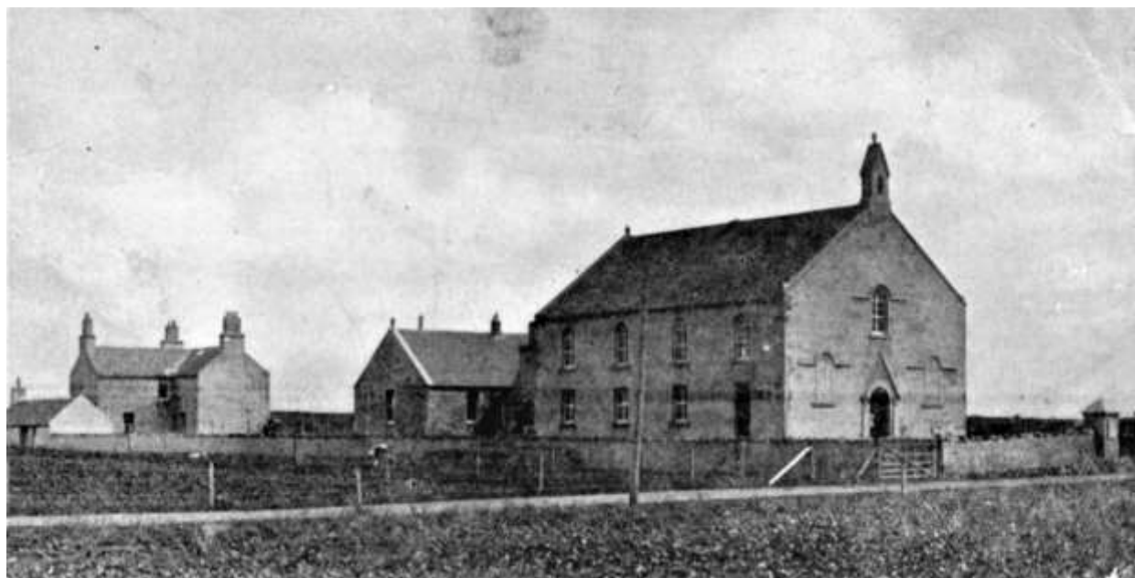
The old United Free Church, still in use in early 1951 but demolished to make way for the new Moncur Memorial Church.
