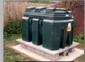
Oil Tank Installation
